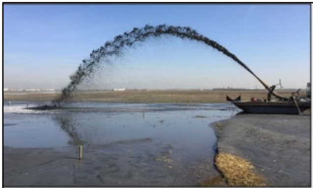
Example of beneficial reuse – dredged sediment application to raise marsh elevation. Credit: San Mateo County.
