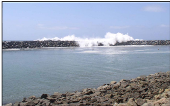
Dana Point Harbor breakwater. Credit: Dana Point Harbor
