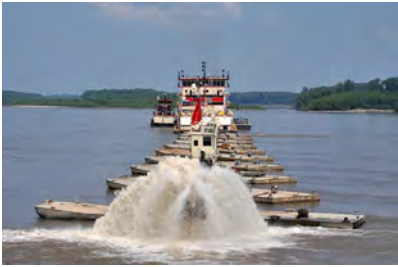
Sediment "Recharge" via Dredging
