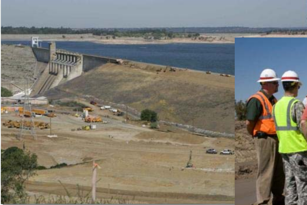
Construction continues on the new spillway at Folsom Dam.
